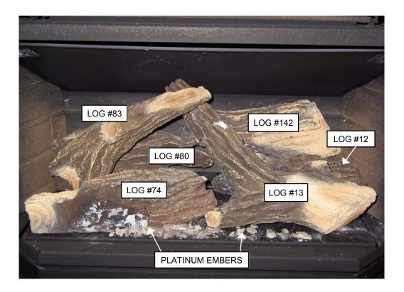
**NOTE:** Installing the ceramic logs in any other position other than shown will result in flame impingement causing sooting of the logs, brick liner and ceramic glass viewing area.
